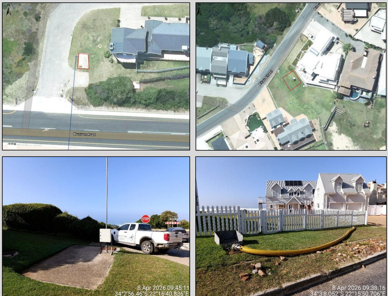
Figure 3: Maps & Photographs of the Eekhorning Street Conservancy Tank (Left) and Bitou Street Conservancy Tank (Right).
