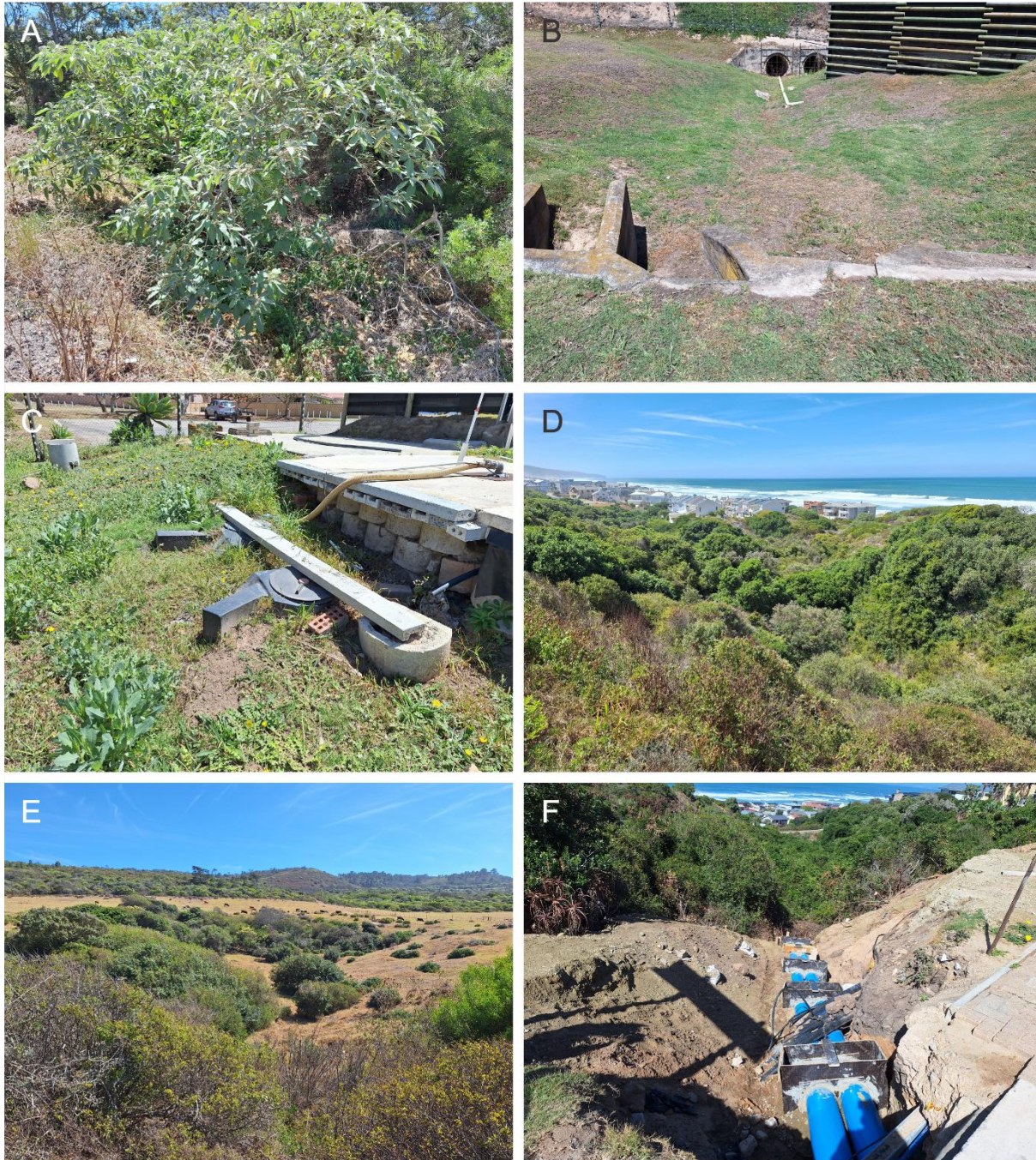
Figure 20: A – Alien invasive Solanum mauritianum (Bugweed) within the mapped watercourse at the first crossing, B – Culverts aligned with the watercourse at the first crossing with overflow pipe of conservancy tanks, C – Conservancy tanks adjacent to the west of the mapped watercourse, D – A view of the flow path at the second crossing towards the south, E – A view of the flow path at the third crossing towards the north showing the agricultural field, F – A view of the flow path at the third crossing towards the south showing the exposed existing infrastructure in sandy soil.
