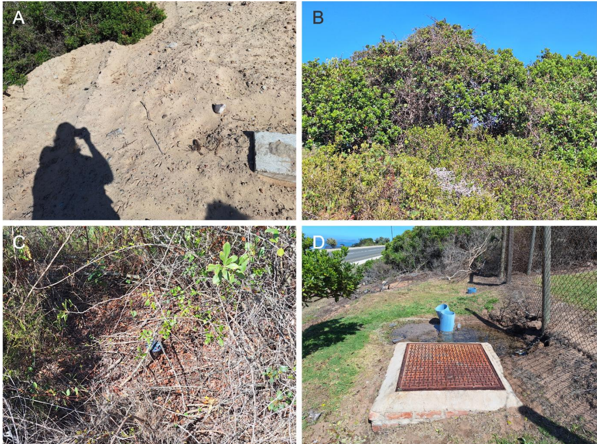
Figure 19: A – Sandy soil in the location of the proposed sewer line, B – General vegetation in the area, C – Evidence of alien clearing, D – Leaking potable water pipe.
