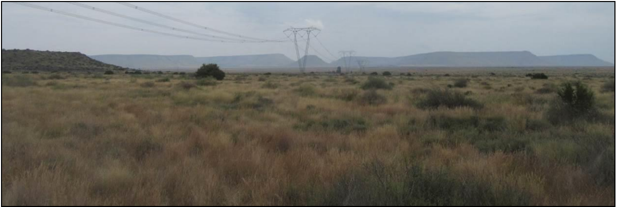
Photograph 3.4: 765 kV line traversing Bas Berg 88/3 to the north of the Kareekloof site
