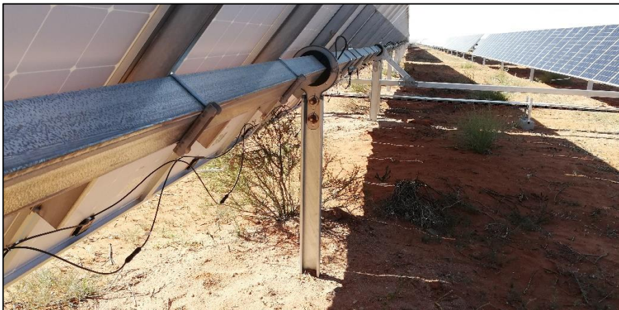
Figure 9: Completed ramming and assembly showing vegetation remaining intact beneath the modules.
