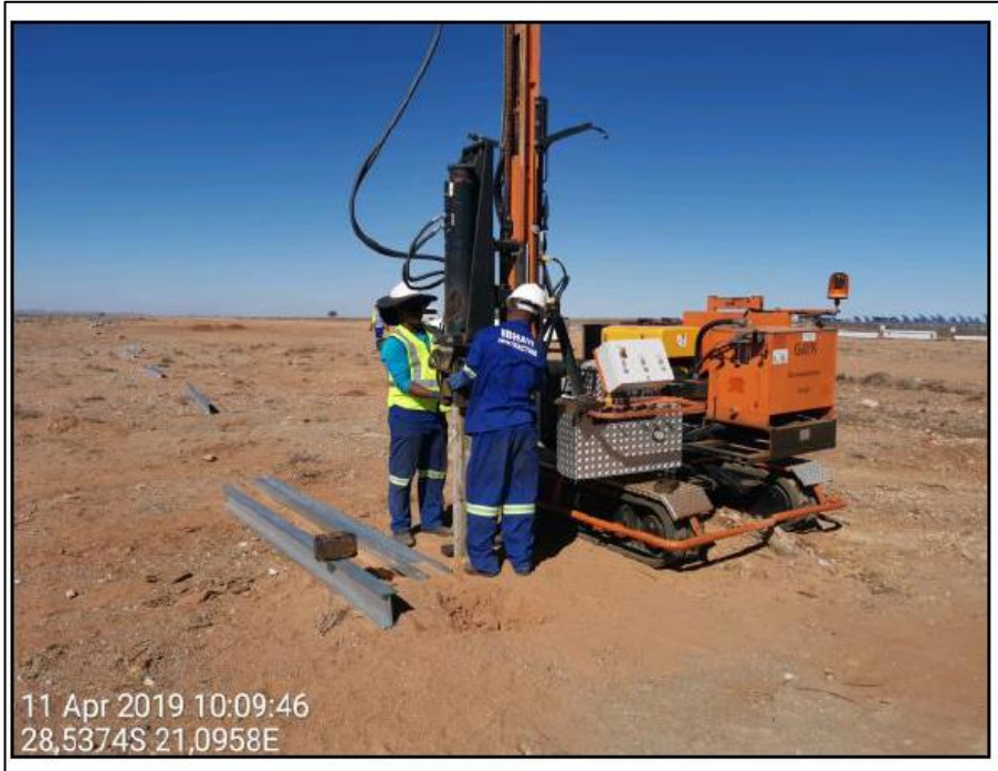
Figure 8: Ramming of steel piles into the pre-drilled / backfilled holes.
