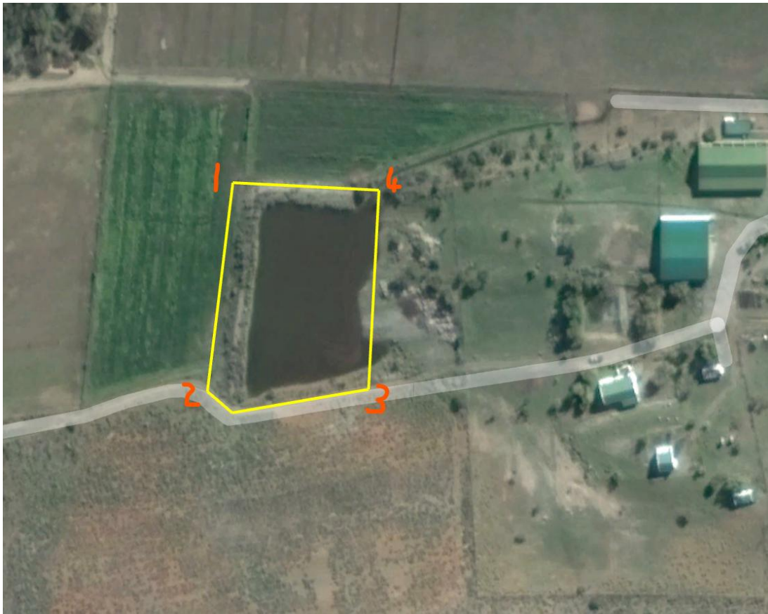
Figure 1: Existing irrigation dam to be re-purposed as runoff effluent dam for feedlot.
