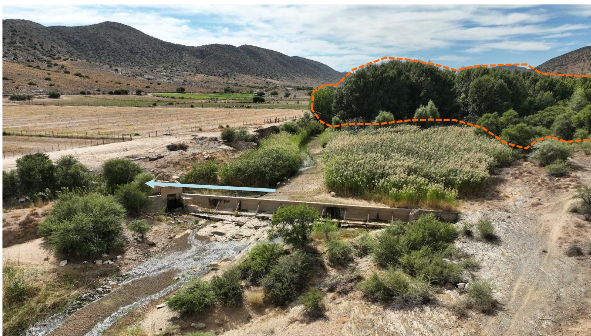
Figure 17. Weir approximately 90m upstream of the road crossing which diverts water via a furrow (blue arrow) to the Stilbaai Dam. Orange = dense invasion of Populus sp.
