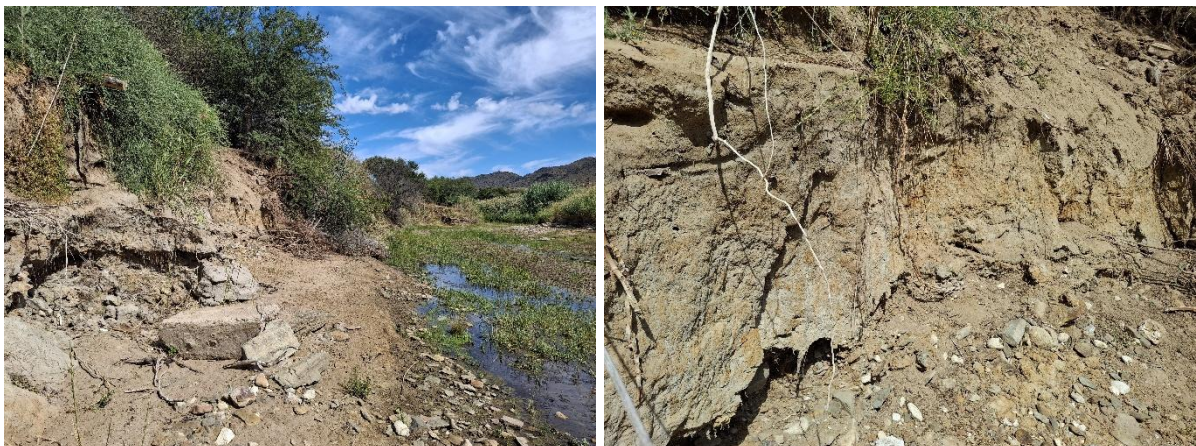
Figure 16. Bank erosion downstream of the road crossing indicating high levels of soil mottling consistent with wetland conditions.
