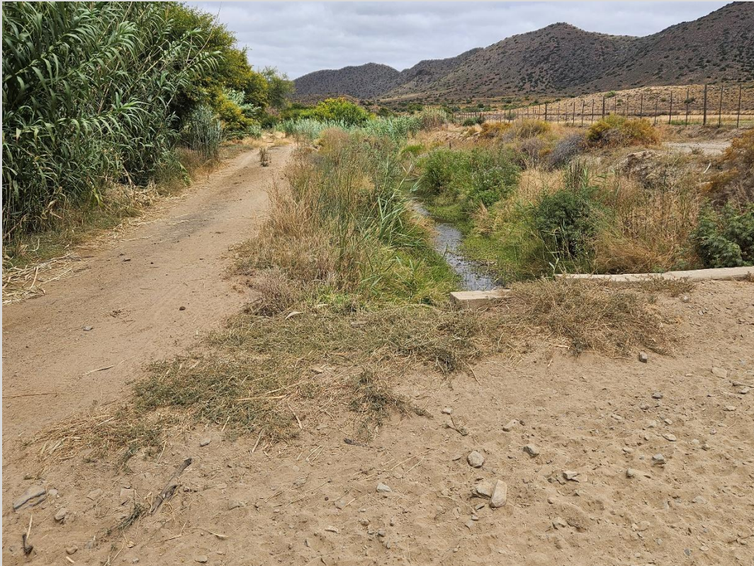
Figure 9: Existing structure over the Jan Rolms River to be upgraded.
