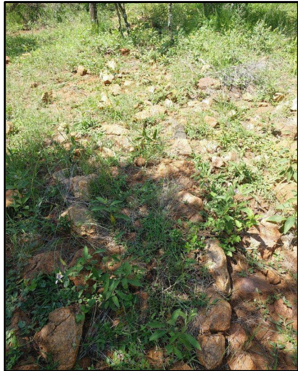
Figure 7.9. General view of the stone packed wall foundation at RG101.
