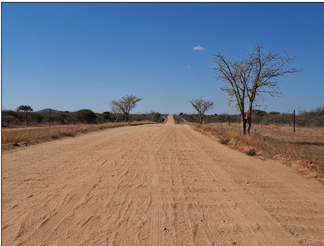
Photograph 3.4: View along Mogwadi/Bottelier Road looking west
