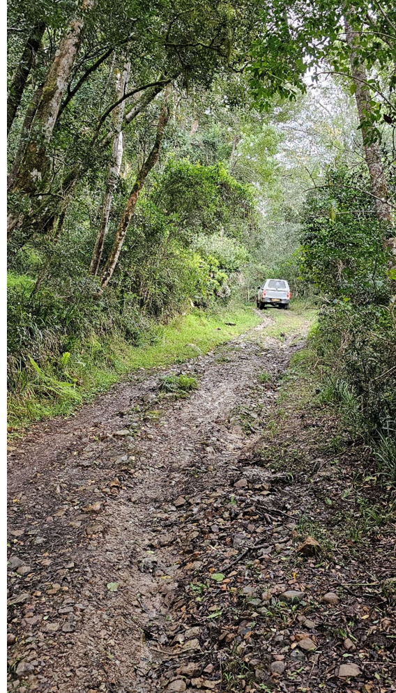
Figure 19: Photo 10, the surface remains uneven and stony, with loose rocks and exposed aggregate further hindering access.
